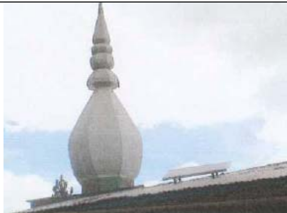
Solar module mounted on top of a mosque as part of solar home system
