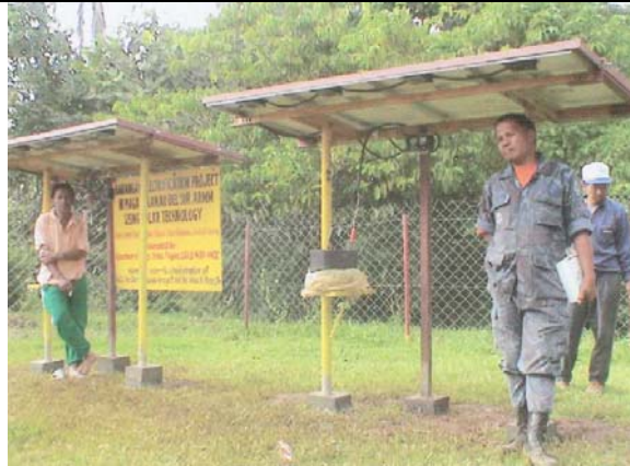
Two of 4 channel of the solar battery charging station
