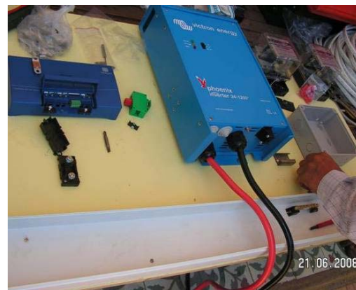
Installation of inverter and charge controller
