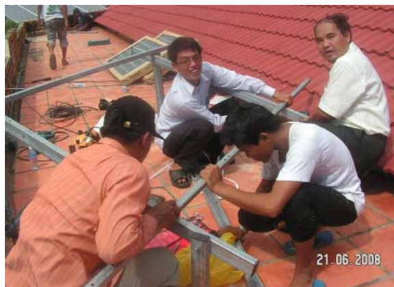
Installation on the office roof
