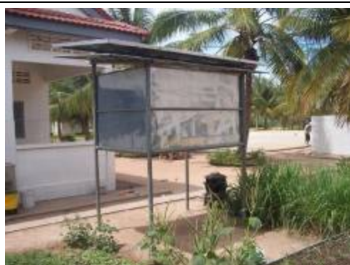
Moved panel from its first position to a shadow-free location
